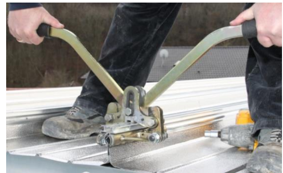
Figure 5: Preparatory seaming with hand seaming tool
