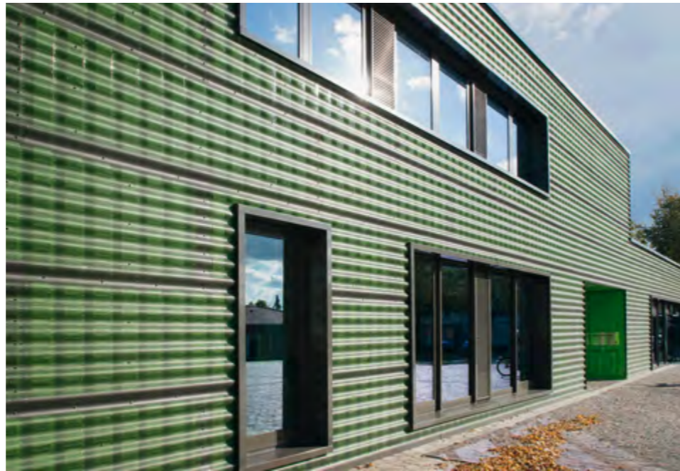
Family Centre SOS Kinderdorf e.V. // Germany Architecture: Thalen Consult, Maike Winter Photo: S + T Fassaden GmbH
