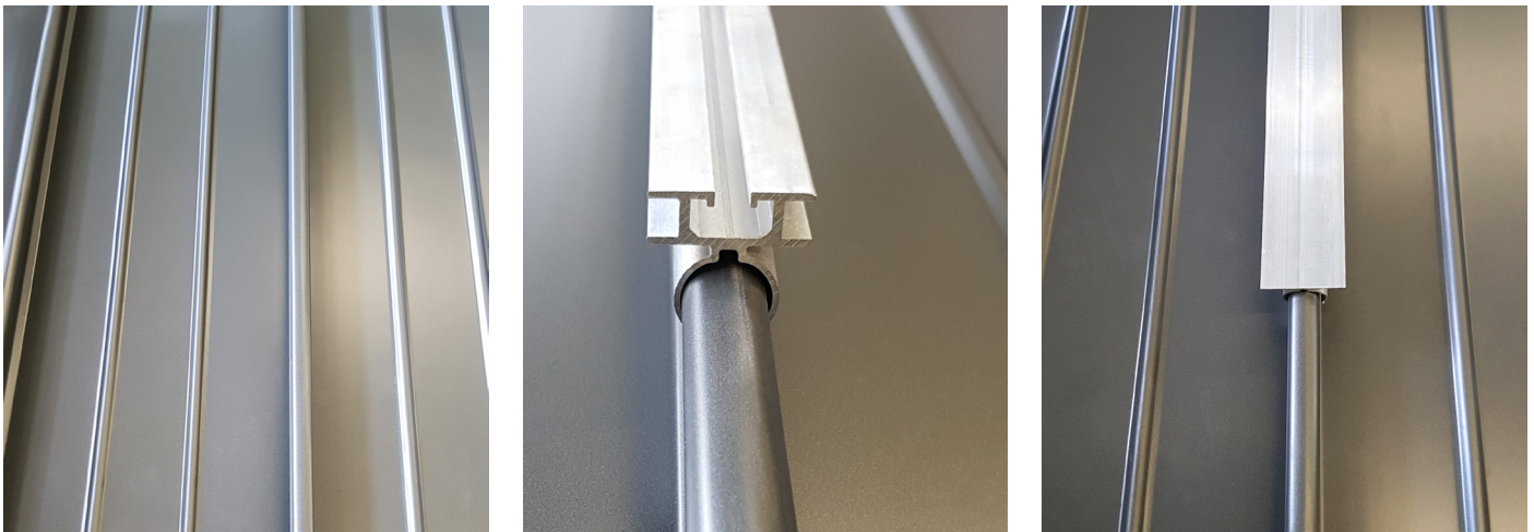
1. Ready-seamed BEMO-Standing seam 2. Attaching Akkord-rails (left) or Top-rails (right)
