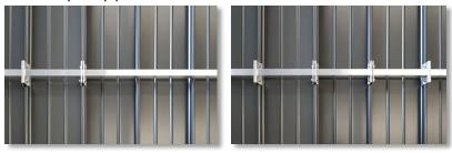
Step 3: Tighten the screws of the clamps with 35 Nm.
