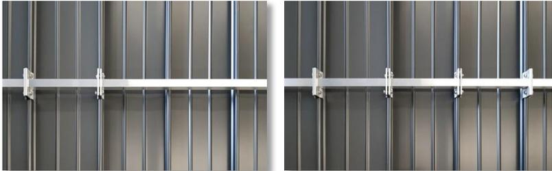
**Step 3:** Tighten the screws of the clamps with 35 Nm.
