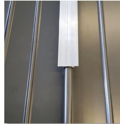
**Step 2:** The hand seaming tool is placed on the profile and seamed with the BEMO standing seam profile by pressing the grip pieces apart. This process is done over approximately the first 30 cm of the rails.
