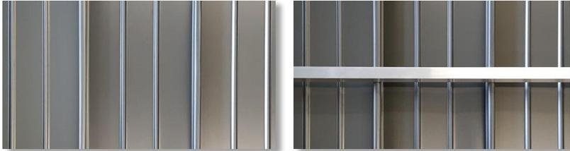
**Step 2:** The fixing clamps are screwed on and slipped over the square pipe at each seam.
