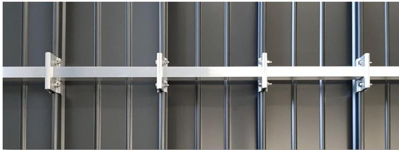
**Step 4:** The snow stoppers are inserted over the square tube at each bead of the BEMO standing seam sheets, aligned on the ridge side.
